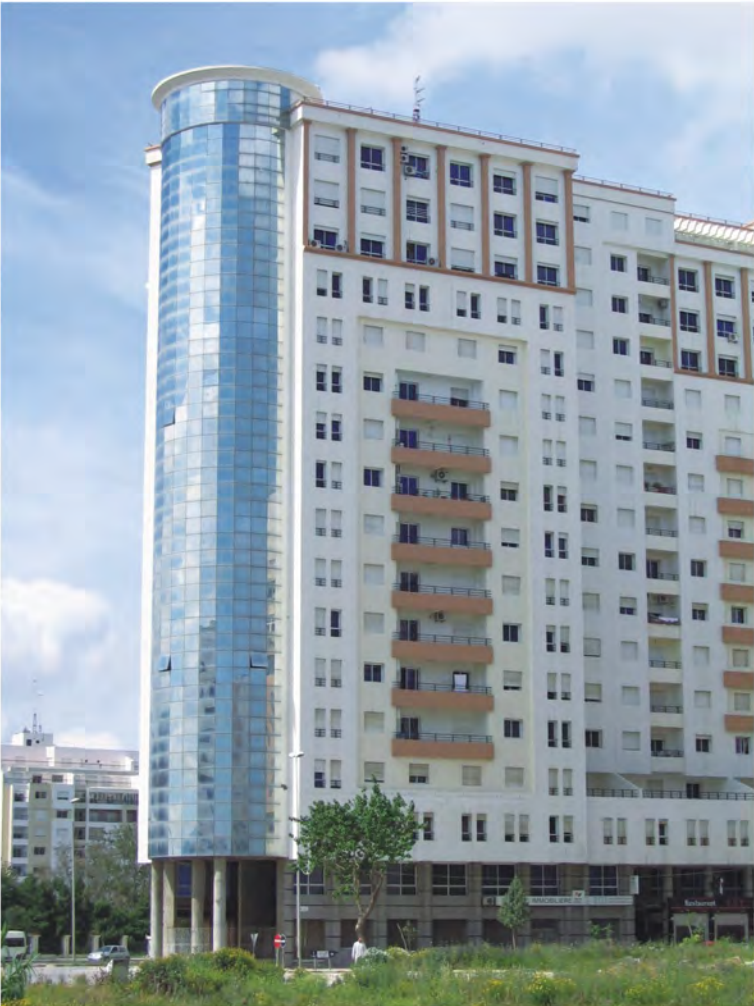
Residential Building Soulainman, Tanger, Morocco
